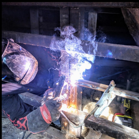
John Norman Welding on the Clough Cave gate. Photo Credit: Steven Johnson
